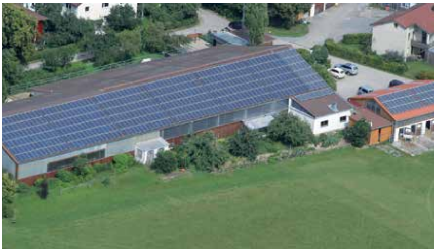
Gäufelden-Nebringen - Germany System: 31,85 kW | SpeedRail
